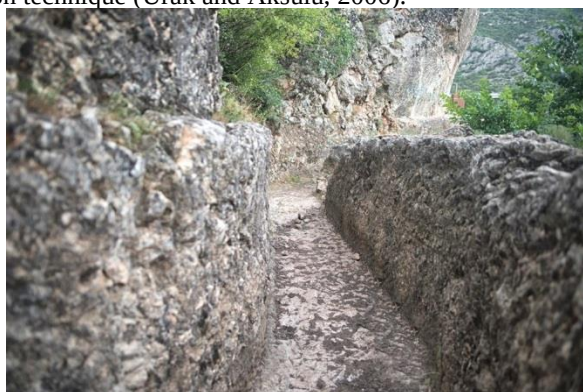
Photo 1. A Section from the Ferhat Water Canal-I.
